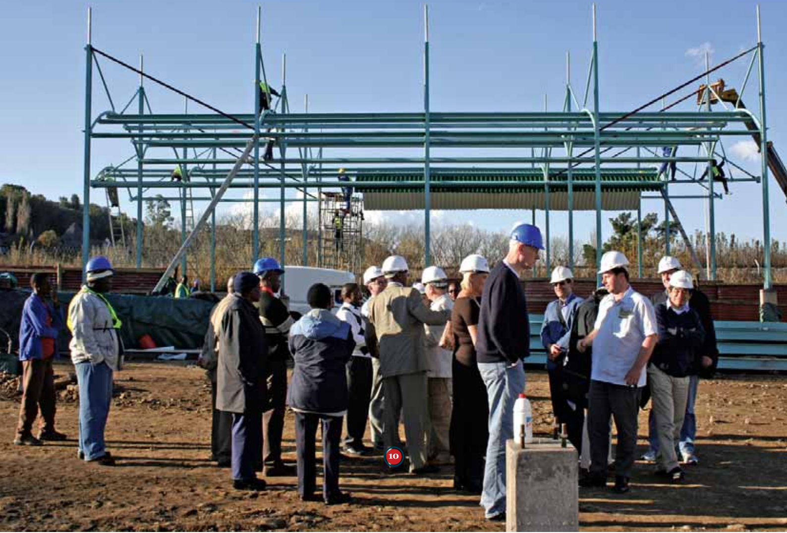
The WCO delegation touring the construction site at Maseru Bridge.
